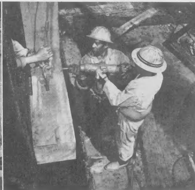
BEFORE DOWELS cover the openings, the area must be drilled to size, far left, and the bolt covered, left. The twelve-by-twelve-inch timbers are picked up and positioned by a crane after the bolt and dowel holes have been drilled. Holes are visible in the timber above.
